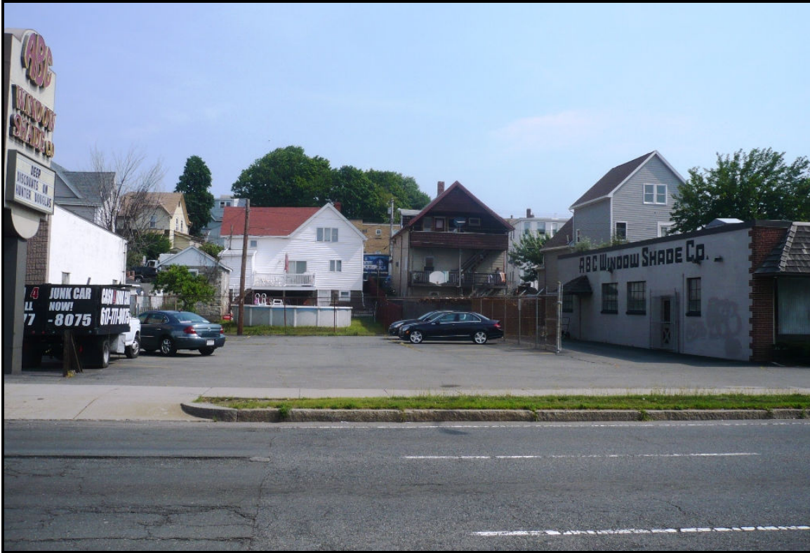
Parking Lot & Pylon Sign (left side of photo)
