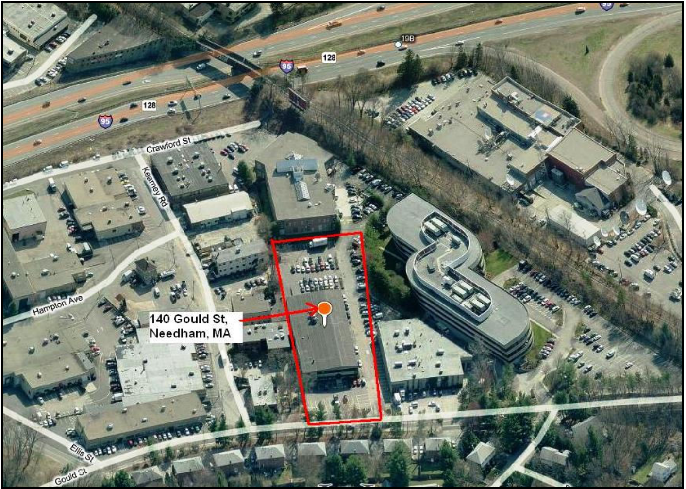
Aerial View from the front of the building on Gould Street
