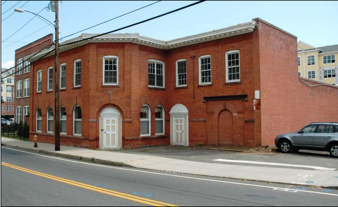
Partial Front View of the Subject
