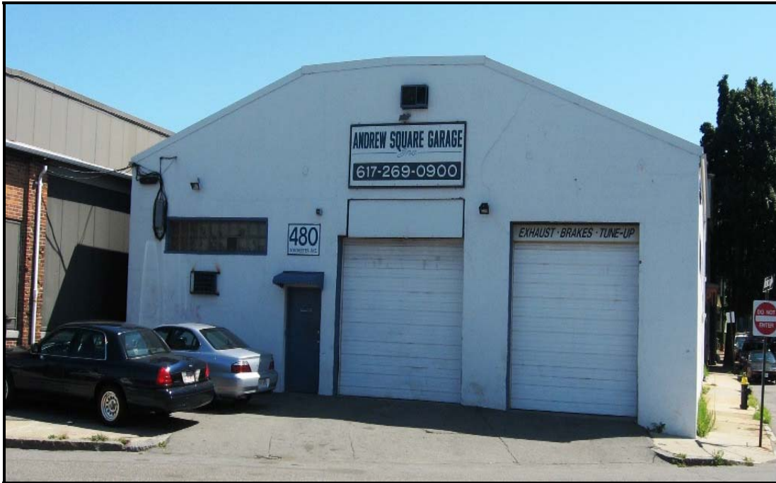
Two Overhead Doors on Dorchester Avenue
