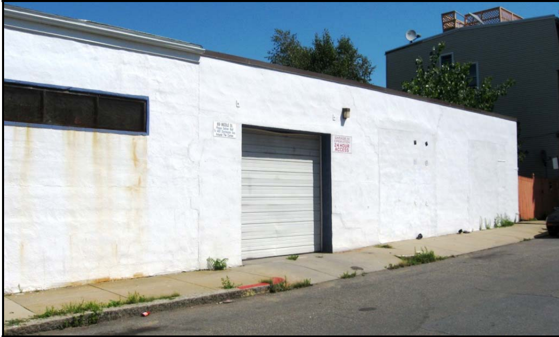
One Overhead Door on Middle Street
